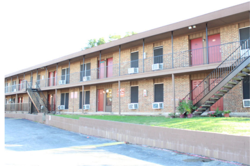
66 Unit Property in Dallas, TX July 2018
