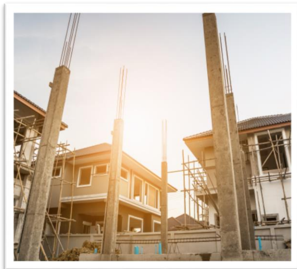
After a renovation or addition
